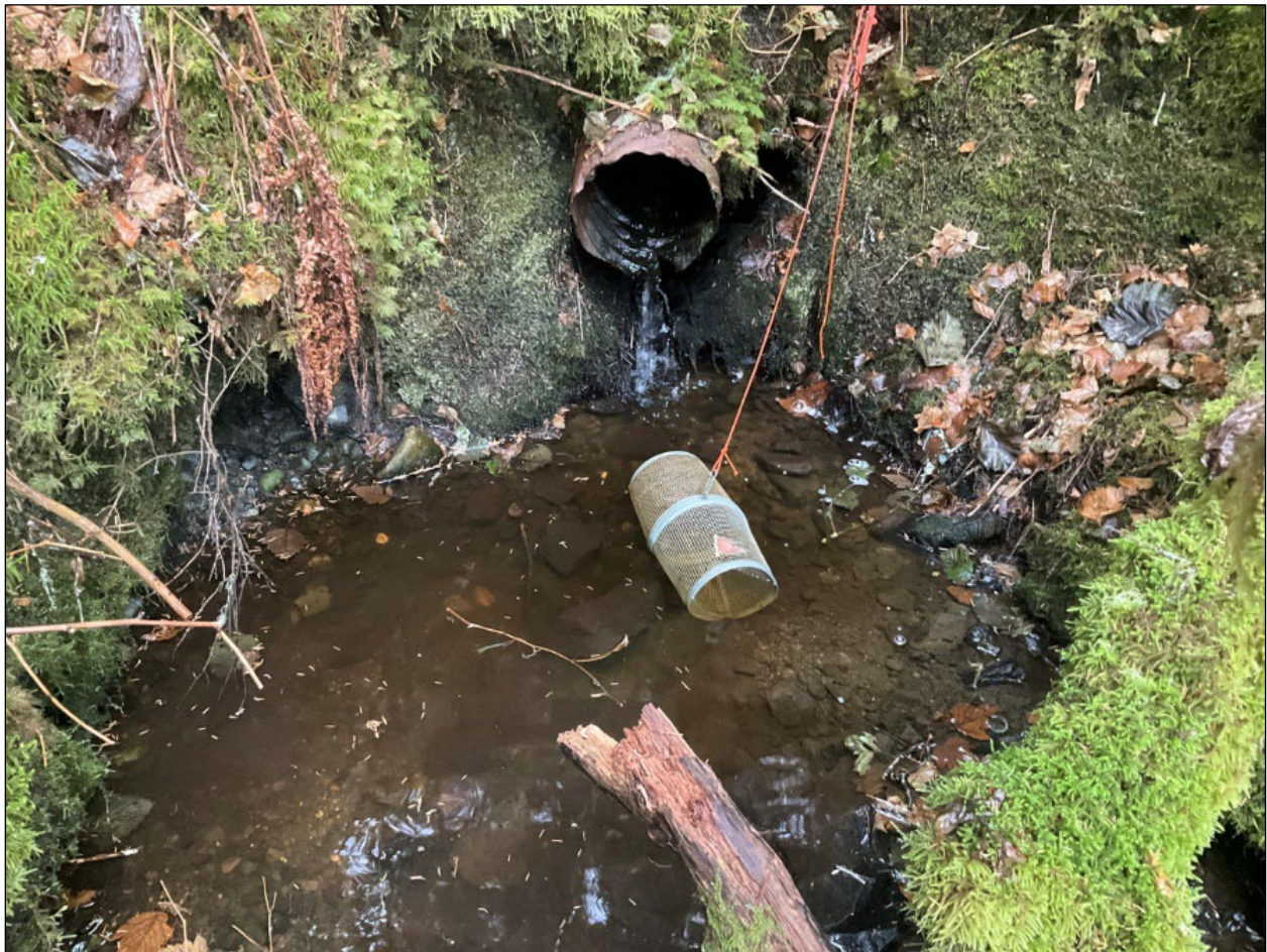
Figure 1.–Culvert outlet at waypoint 1095.
